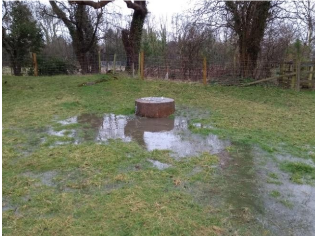
Sewer flooding in sheep field east of Church Lane Storm Henk January 2025
