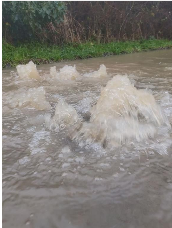
Corner Allenby Cres showing surcharging sewer pumped from Utterby pumping station leading to sewage spills following heavy rainfall
