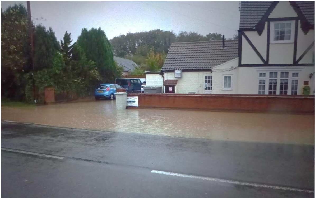
Surface water flooding from overflow at the Dock pooling at low point outside Fotherby Care Home, Louth Road. Some ingress of flood water into kitchen (Storm Babet Oct 23)
