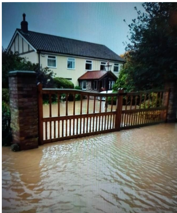
Church Lane East - flooding in the grounds of The Laurels, Church Lane (Storm Babet Oct 23)
