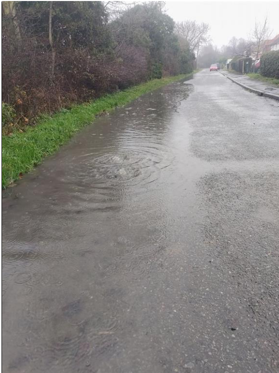
Corner of Allenby Crescent showing surcharging sewer pumped from Utterby pumping station, leading to sewage spills following heavy rainfall.
