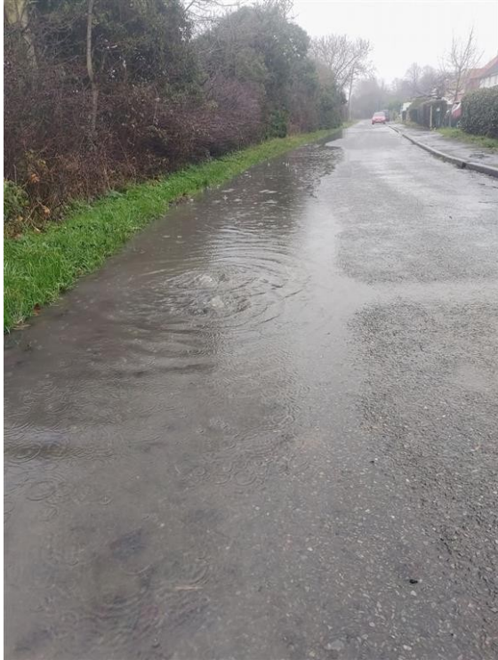
Corner Allenby Cres showing surcharging sewer pumped from Utterby pumping station leading to sewage spills following heavy rainfall
