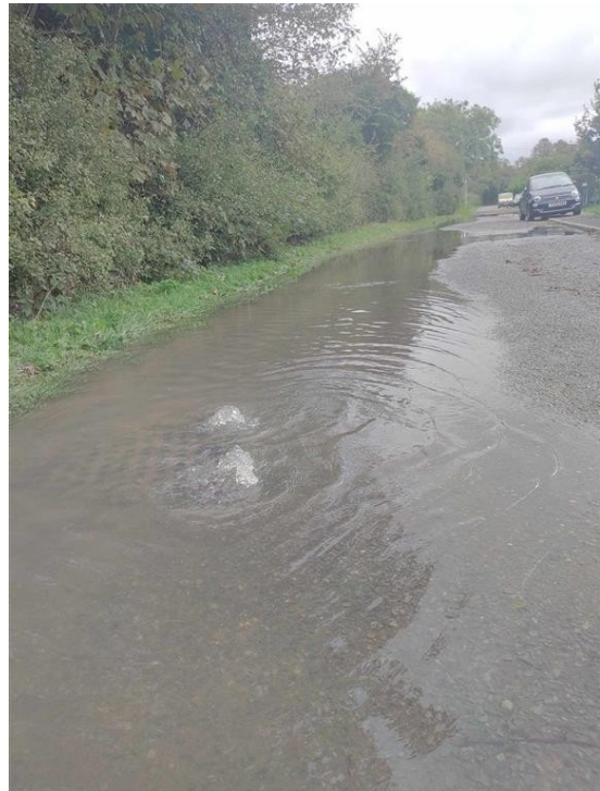
Corner Allenby Cres showing surcharging sewer pumped from Utterby pumping station leading to sewage spills following heavy rainfall
