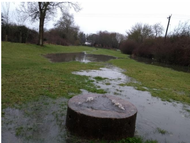
Sewer flooding in sheep field east of Church Lane Storm Henk looking east - January 2025
