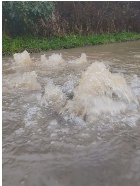
Corner of Allenby Crescent showing surcharging sewer pumped from Utterby pumping station, leading to sewage spills following heavy rainfall.
