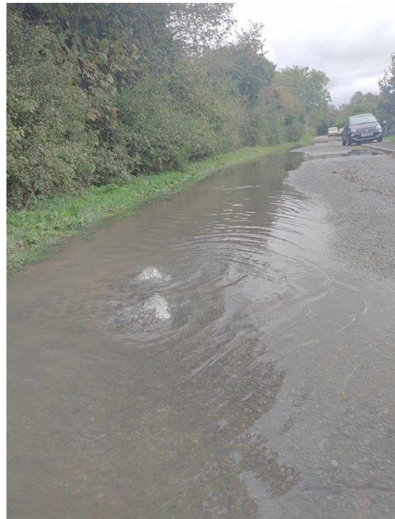
Corner of Allenby Crescent showing surcharging sewer pumped from Utterby pumping station, leading to sewage spills following heavy rainfall.
